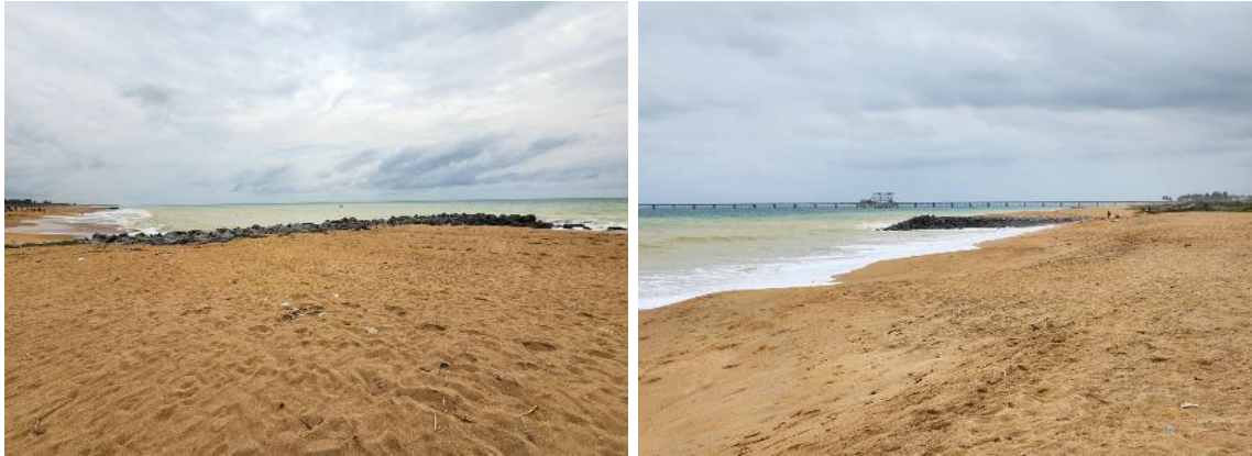
Pictures 16 and 17 – Western and eastern sides of a saturated groyne at Goumou Kopé
