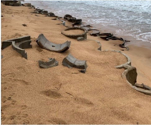
Pictures 10 and 11 – Overturned and broken pipes in Dévikinmé, May 2022 (left) and Tango, November 2022 (right)
