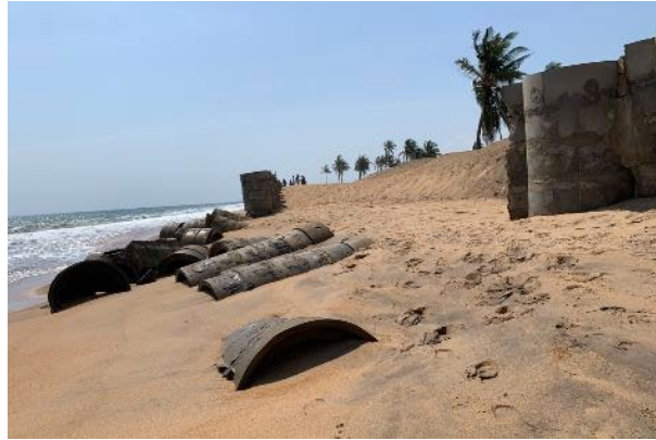
Pictures 10 and 11 – Overturned and broken pipes in Dévikinmé, May 2022 (left) and Tango, November 2022 (right)
